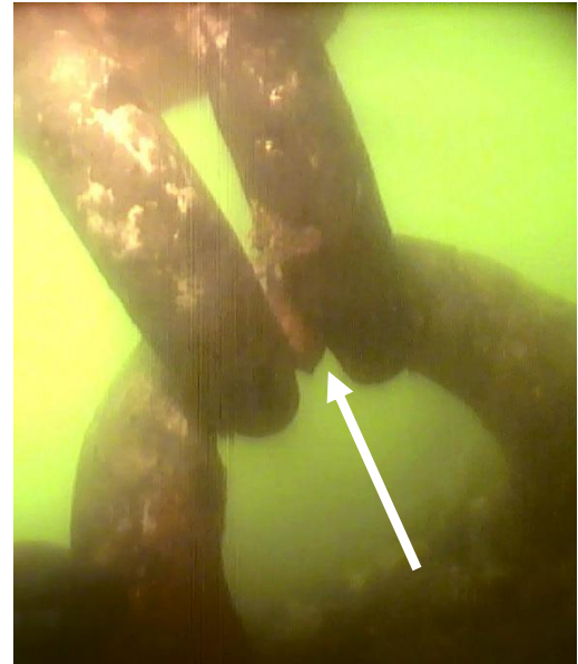
View showing cross section loss on 3" lifting eye
