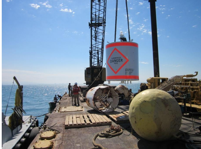
Preparing to install the new top package in 2012
