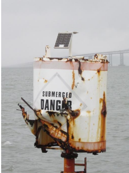
Inshore Marker prior to replacement
